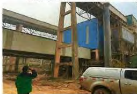
ADA001 中细破车间出料废气排放口A
